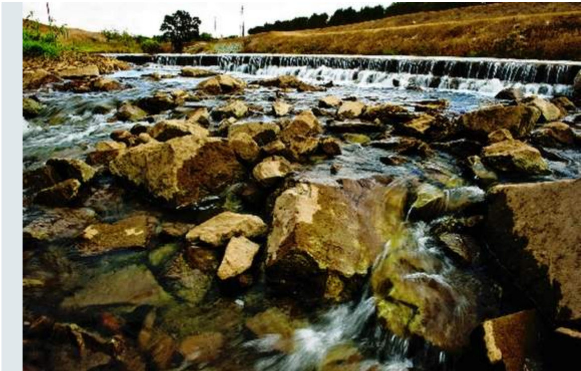
This concrete roadway across Mormon Slough east of Linden is one of four fish barriers that the California Department of Fish and Wildlife have said need to be modified to allow fish to pass more easily.
